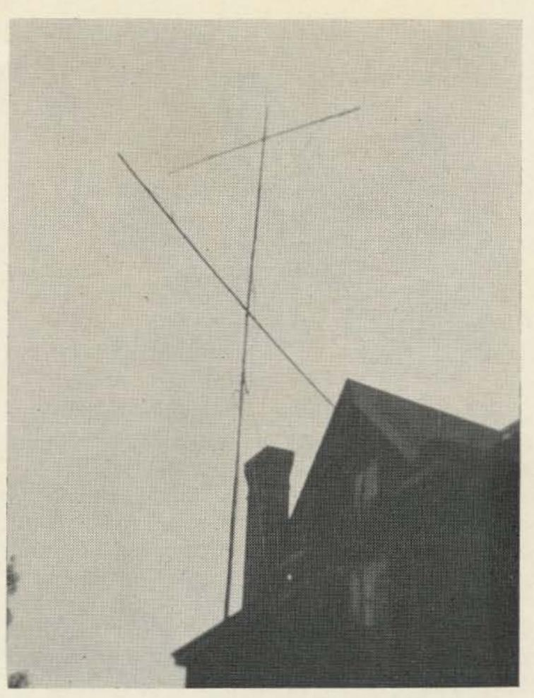
AC4NC KC4USN \* YS1MS \* W5NAX/EAØ \* VQ9HBA VR3L KS6AM UM8FZ 5U7AD ZL4GA JA7AD CN8MB 6Ø1MT UAØKID VK5ZL and dozens of Europeans and So. Americans. (from July 61 to July 62 running 300 watts to homebrew xmtr, average city location) The SWR is 2:1 at 14,000 and 1.3:1 at 14,300 kcs.
